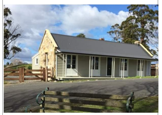
We pulled down the additions from the 1940's onwards and took it back to the 19th century stone core - two walls and two chimneys! The parapets were restored, double posts added to the veranda and new windows and door constructed.
